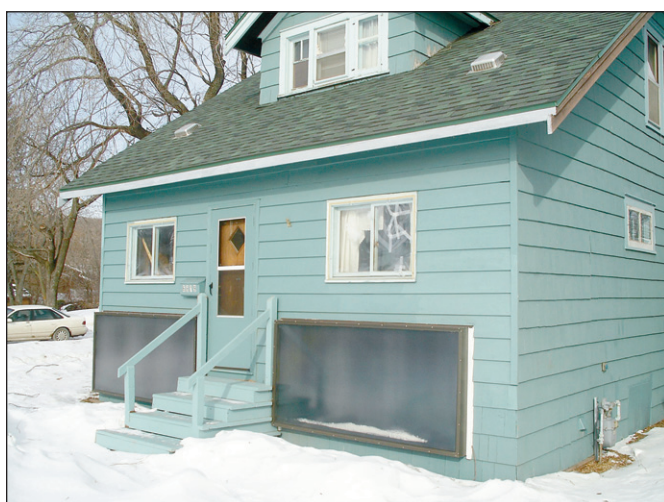
Solar heat can make homes more energy efficient. Solar air heat panels are metal pieces heated by the sun. The solar panels are affordable and work well on sunny days.
